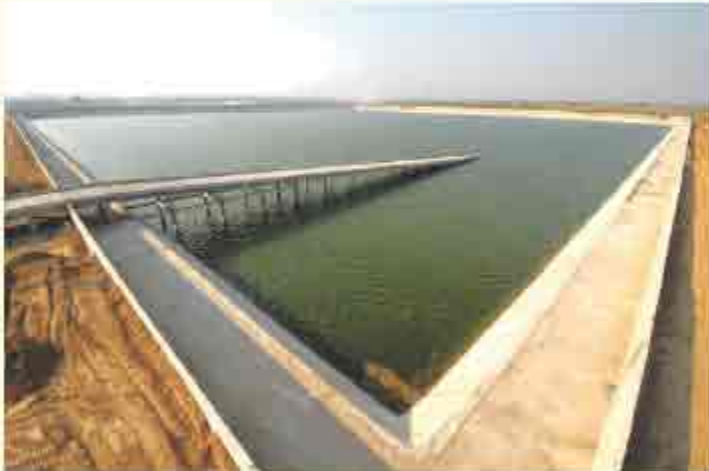
Huda 100 Water Treatment Plant MLD at Gurugram (Haryana)
