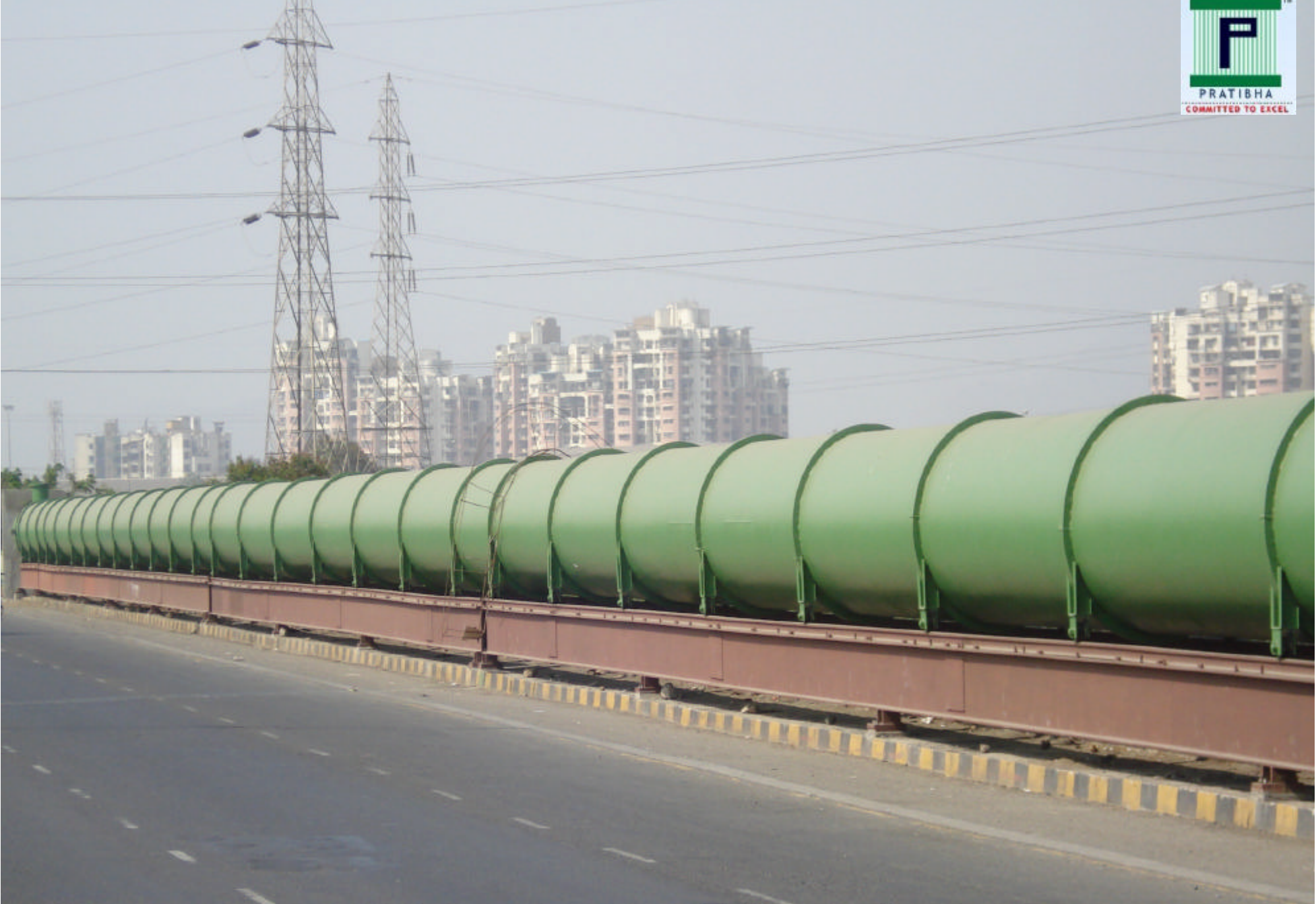
PIPELINE (After Painting)
