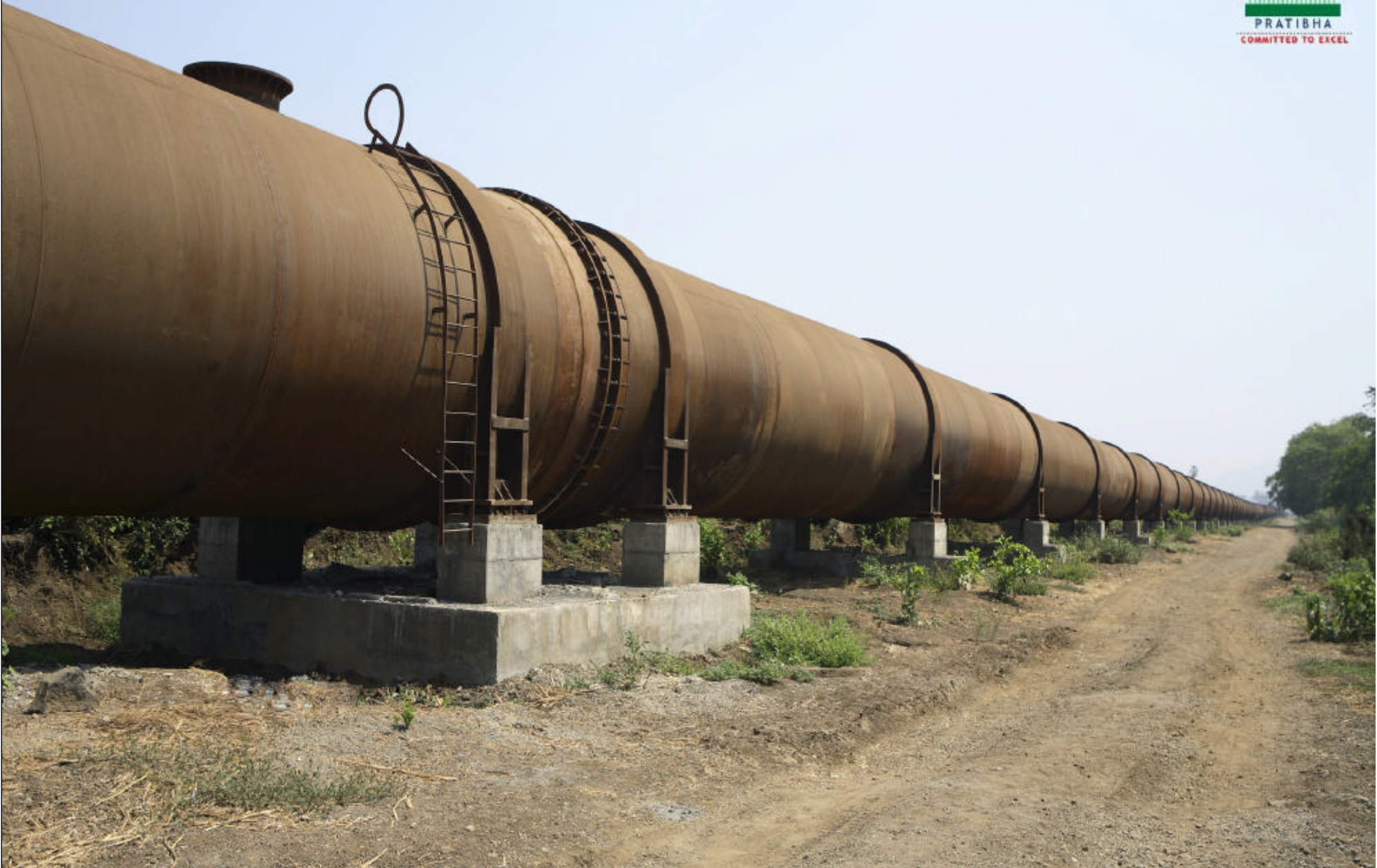
PIPELINE (Before Painting)
