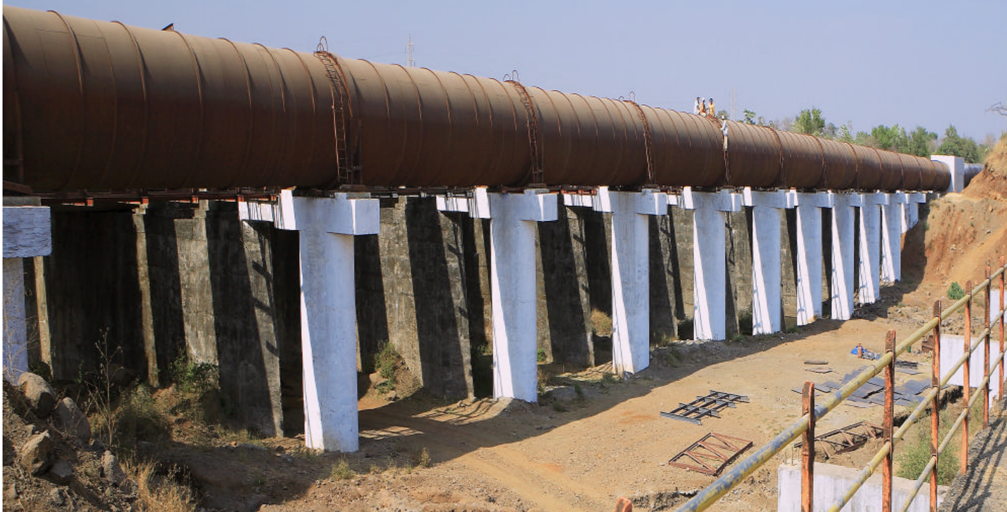
COMPLETED PIPELINE – ABOVE GROUND LEVEL
