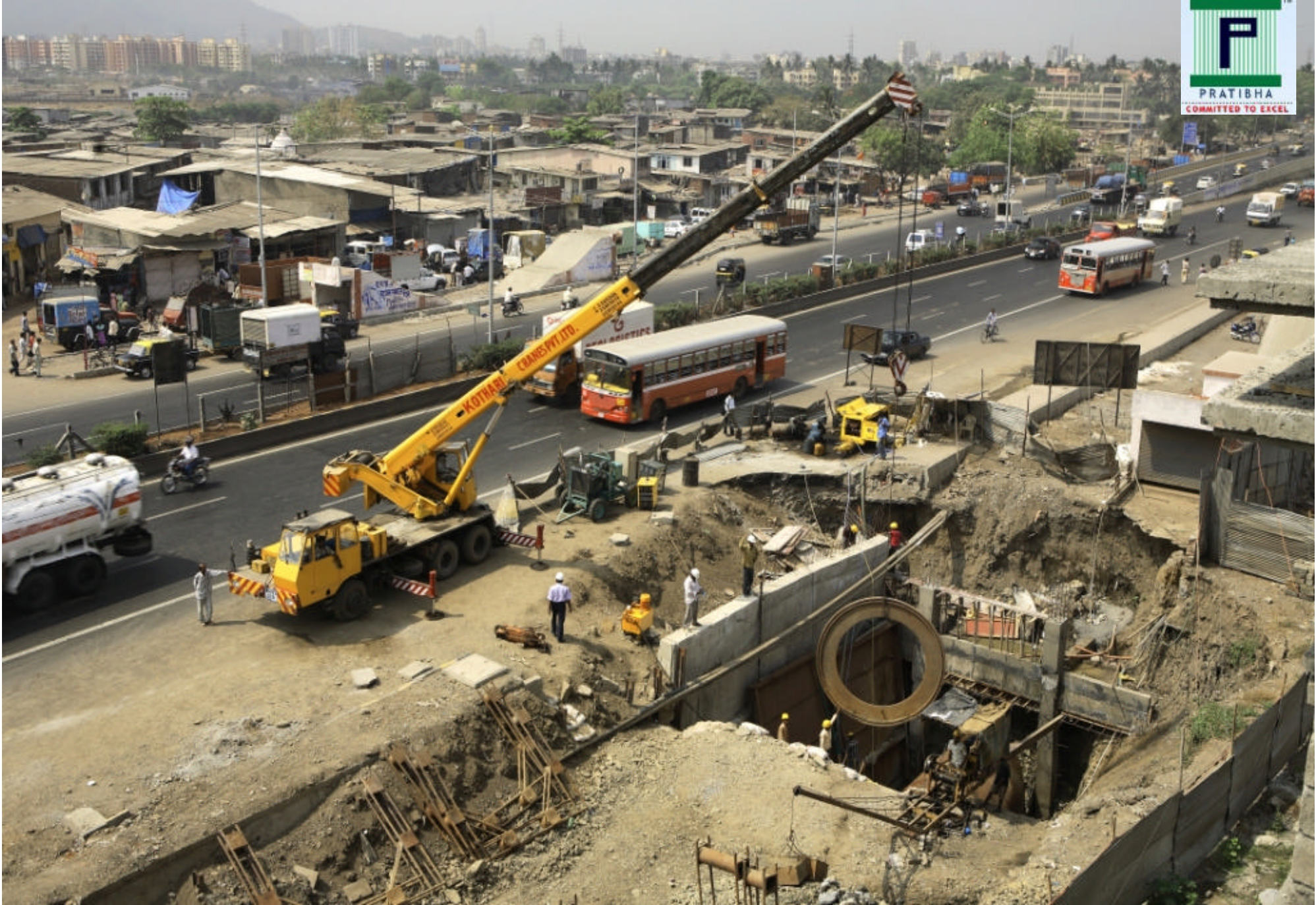
HEAVY MACHINERIES USED AT SITE
