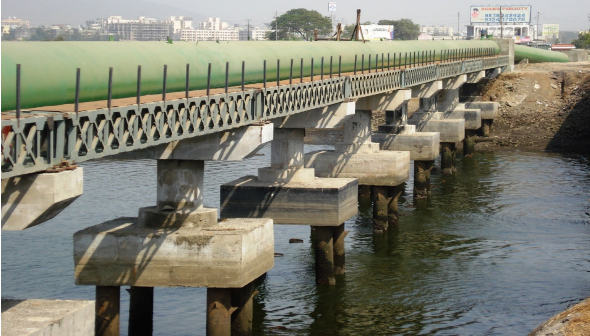
COMPLETED PIPELINE – RIVER CROSSING
