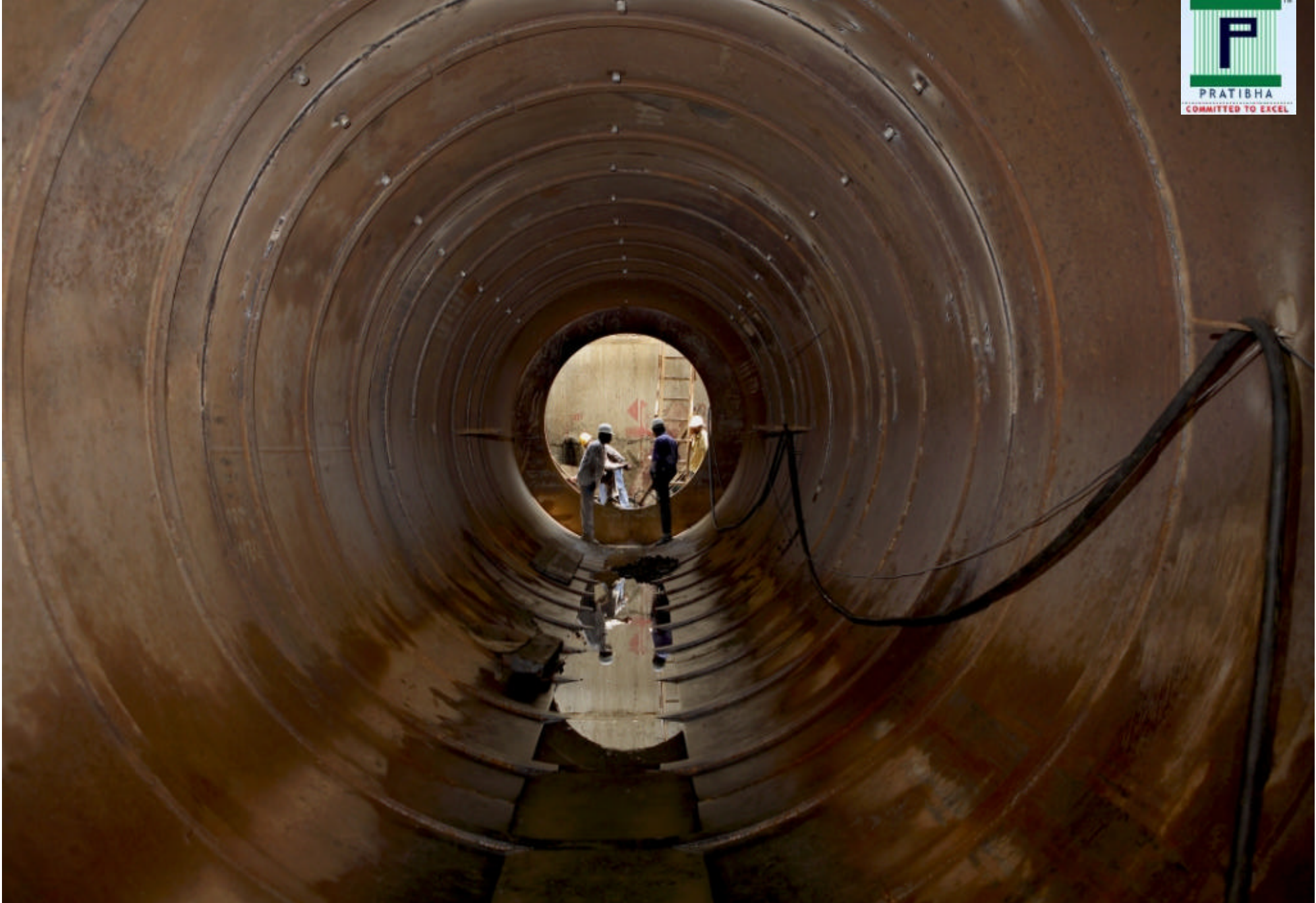
INTERNAL VIEW OF A PIPE
