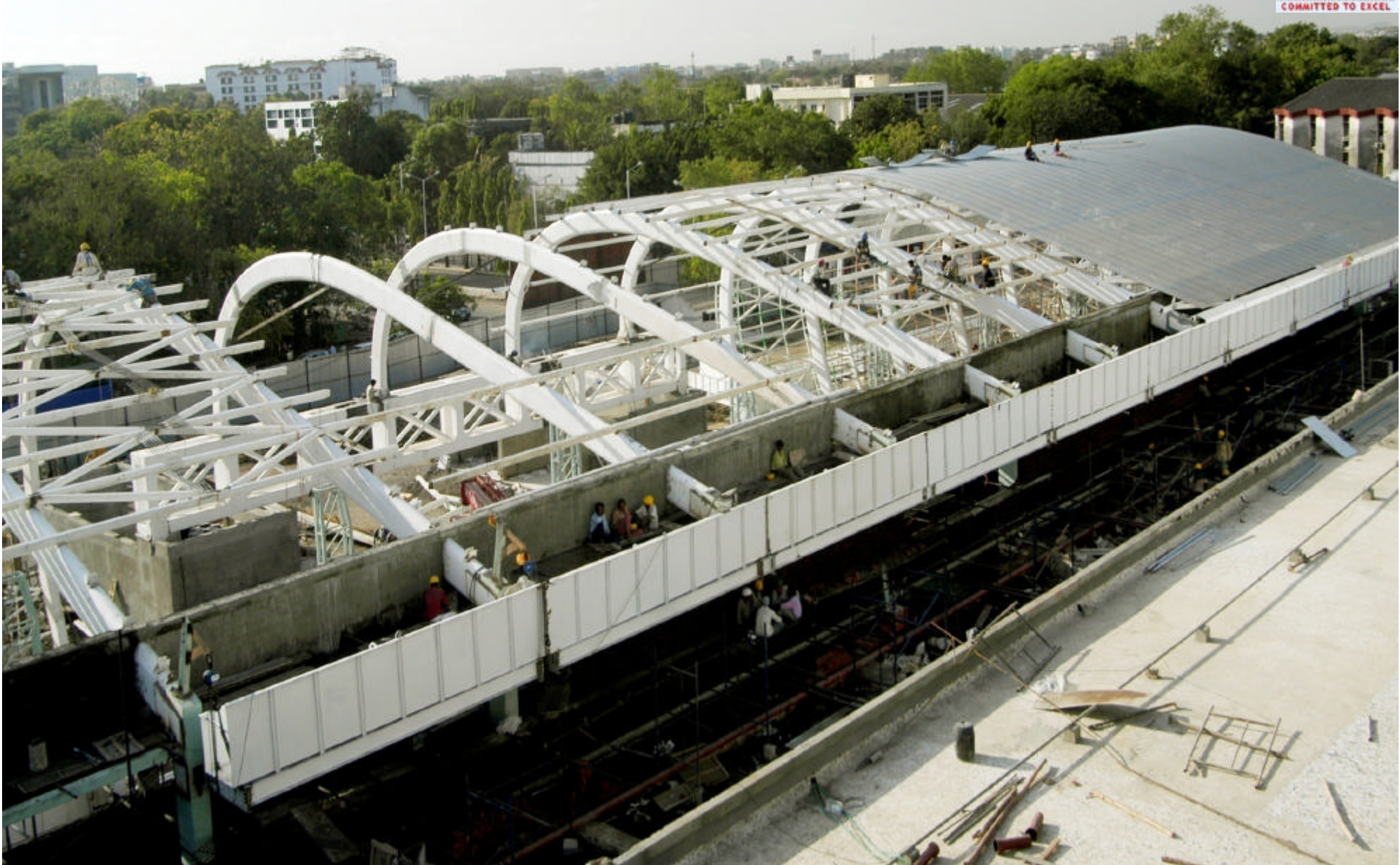
MUMBAI AIRPORT , TERMINAL 1- B
