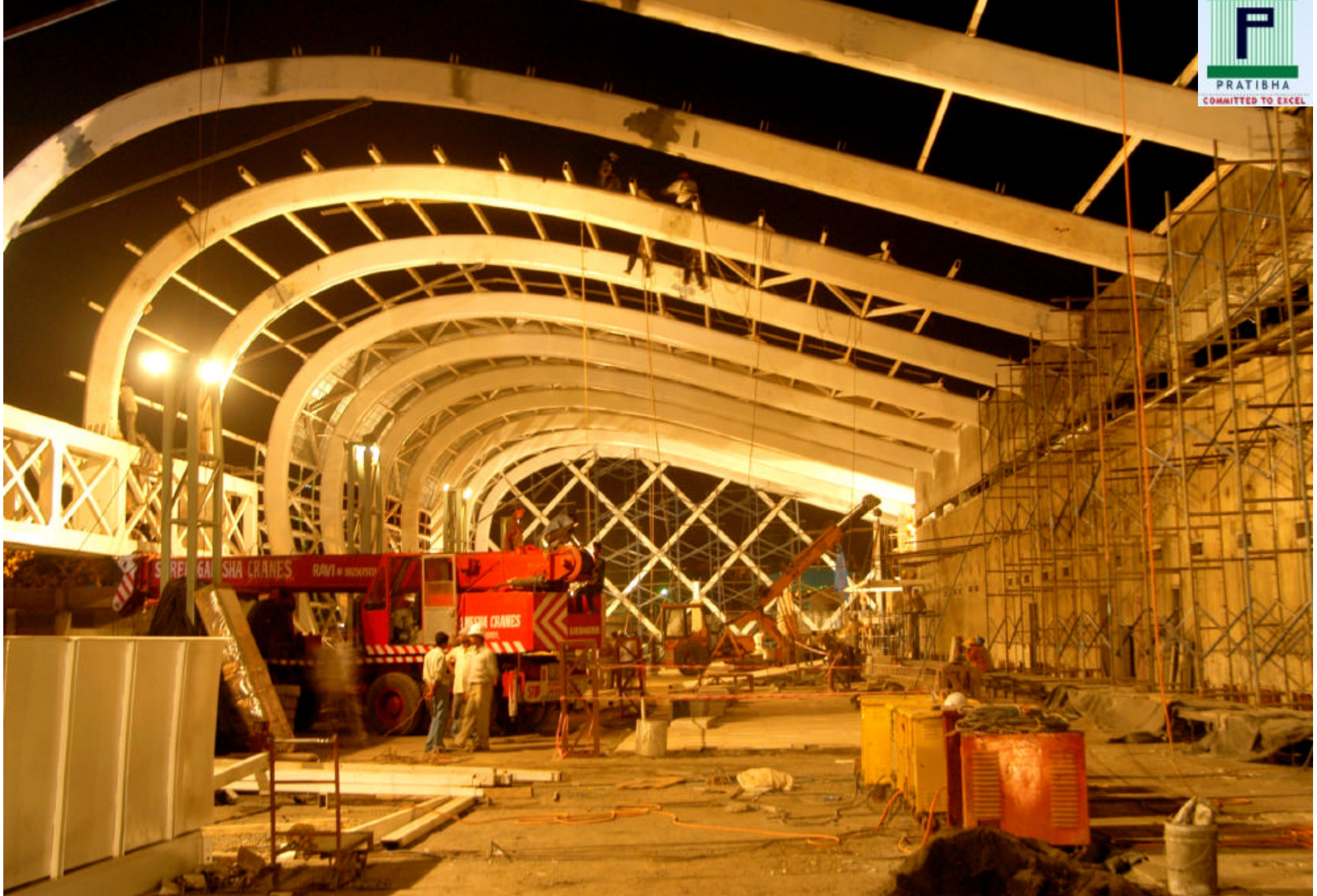
Construction of Mumbai Airport (Terminal 1 B)
