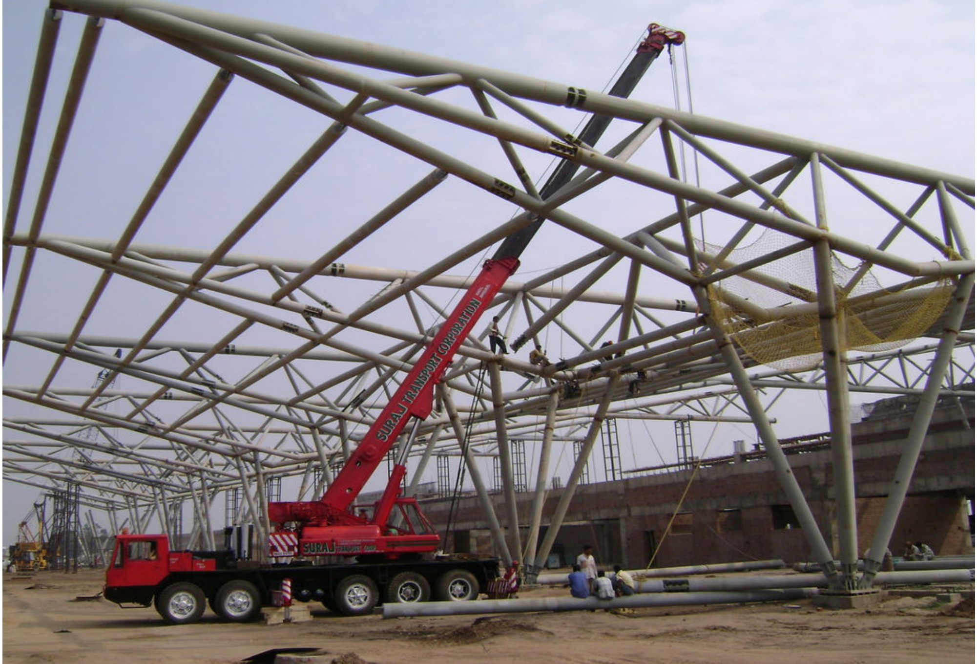
Concourse Purlin Erection
