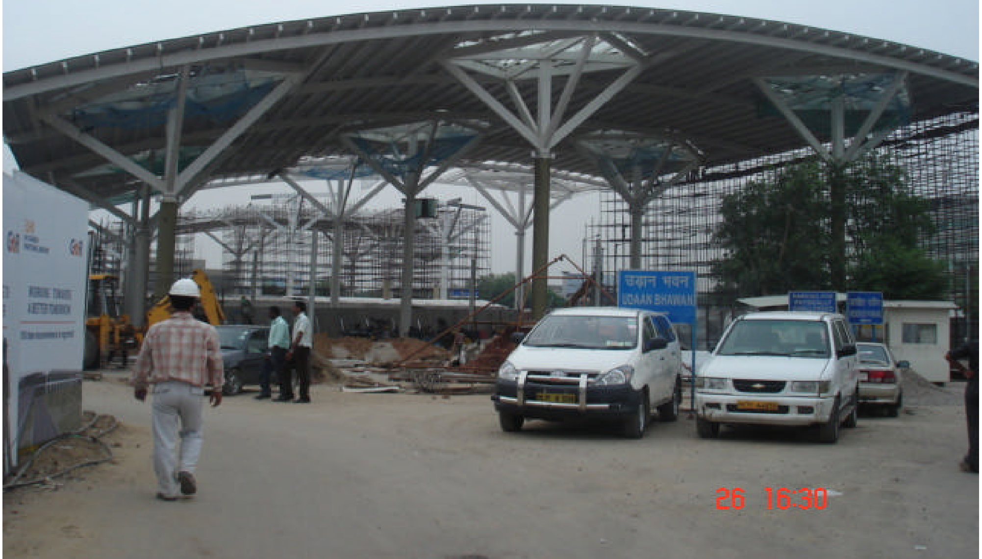
View of the Landside Canopy
